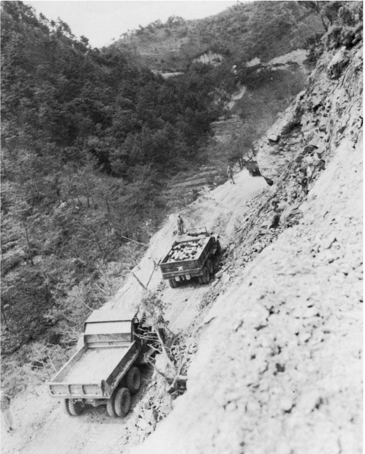
TRUCKS HEADING FOR INJE along newly repaired road, 1 August.
