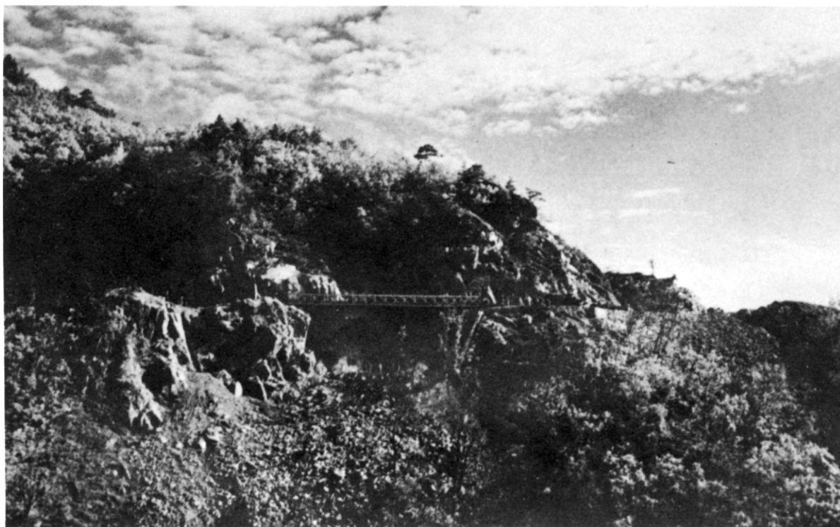
BRIDGE OVER UNDERCUT ON ROAD BETWEEN INJE AND YANGGU, Engineers removed bridge after filling the undercut area to road level.
