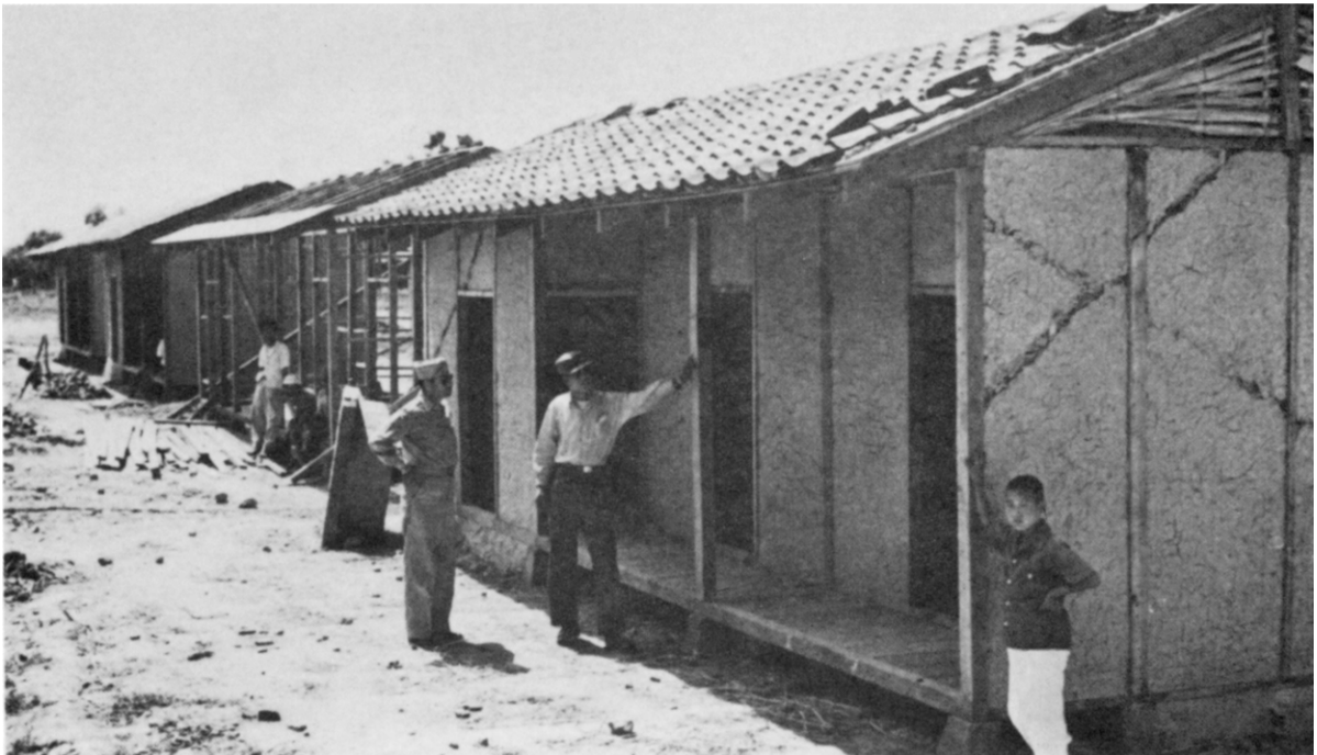
Partially Constructed Family Housing Units, Taeju, July 1952.
