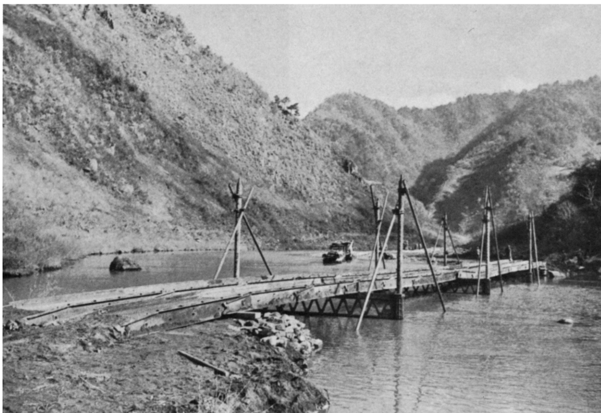
378TH ENGINEER COMBAT BATTALION constructing a treadway bridge across the Pukhan River, ROK 6th Division sector of IX Corps area, November 1951.
