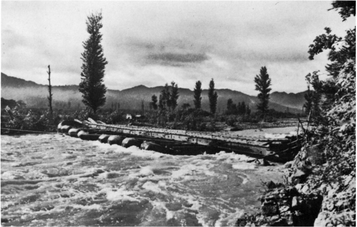
PONTON BRIDGE IN 3D DIVISION SECTOR washed several hundred yards downstream by flash floods. During August heavy torrential rains bogged down lines of communication to the front.
