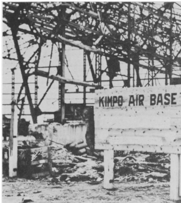
REMAINS OF A HANGAR AND MAINTENANCE SHOP
