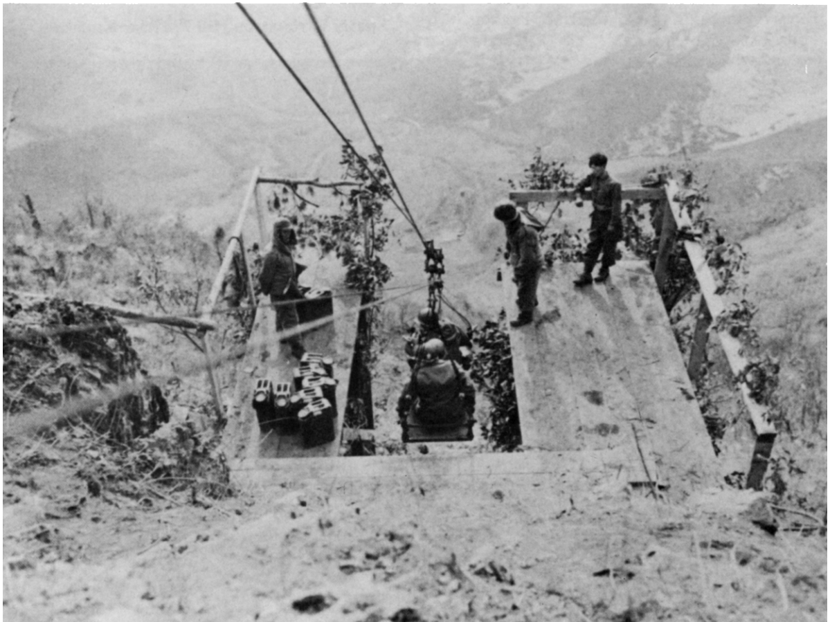
CABLE CAR, built by 3d Engineer Construction Battalion. Starting point is at foot of Hill 770, left; the car nears the platform at the top of the hill, below. Engine from a discarded \frac{3}{4} -ton truck supplied power for the car, which traversed a distance of 1,530 feet from bottom to top. At several stages of its journey the car dangled as much as 200 feet off the ground.
