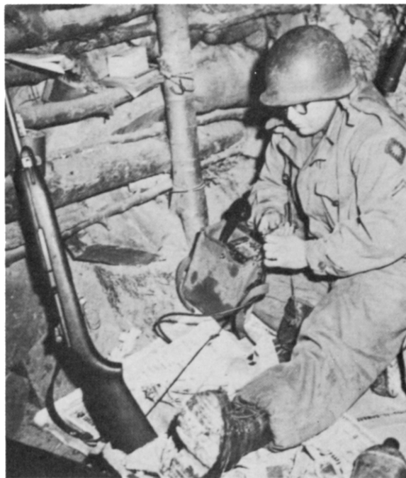
INSTALLING A FIELD TELEPHONE at the 160th Infantry regimental command post.
