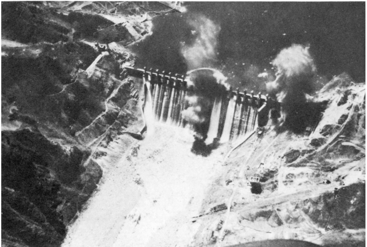
THE HWACH'ON DAM UNDER ATTACK by Navy AD Skyraiders using aerial torpedoes.
