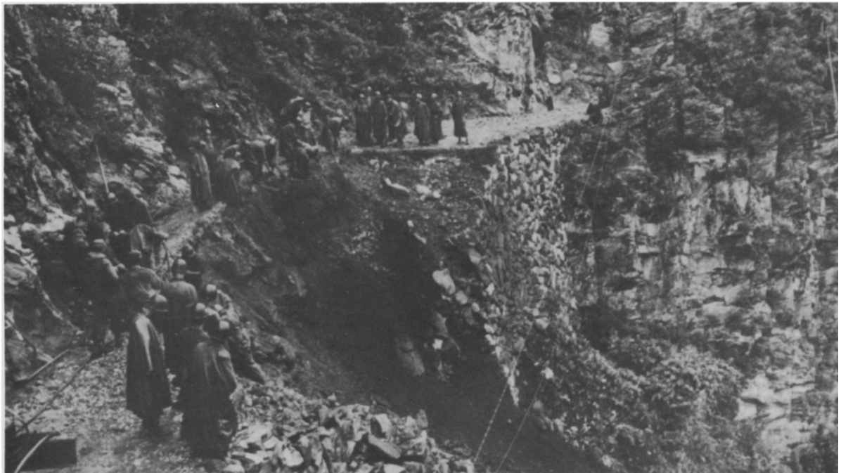
ENGINEERS REPAIRING ROAD DAMAGE caused by heavy rain near Inje, 21 July.
